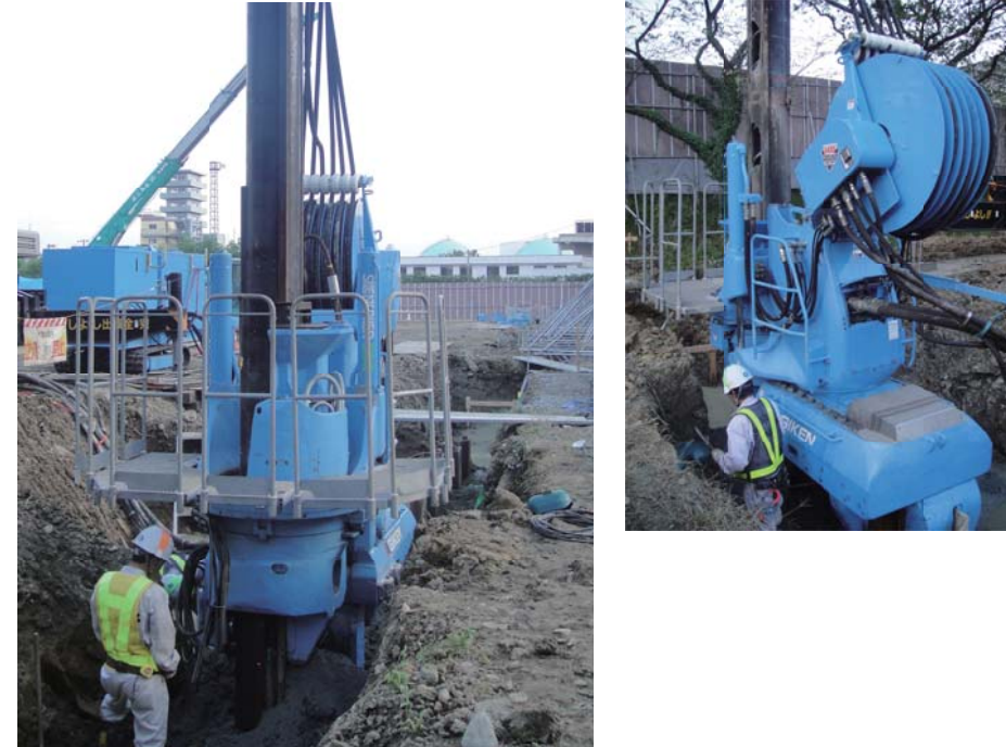
Project : Demolition of Miyagi Prefectural Public Health and Environment Bldg.- Second Phase Location : Sendai City, Miyagi Period : October 2013 ~ November 2013 Silent Piler : F201 Type of Sheet Pile : J Pocket Pile JFESP-4WS, U Sheet Pile SP IIw Pile Length : 4.0 ~ 7.5 m
